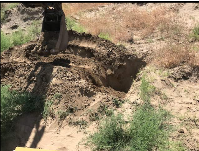
Excavation of test pit TP-2
