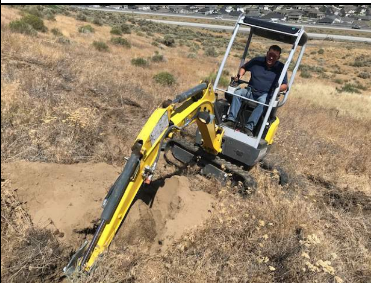
Excavation of test pit TP-3 looking NW
