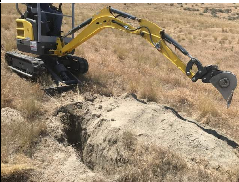
Excavation of test pit TP-7 looking west
