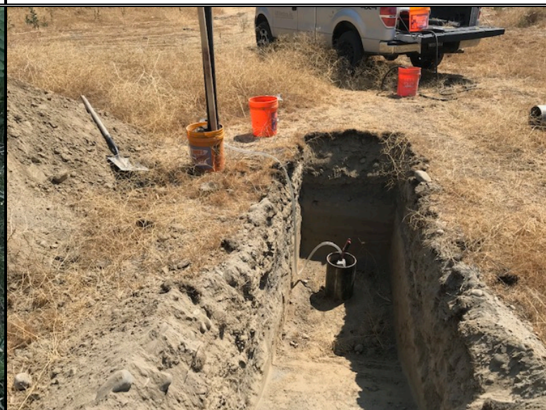
Infiltration test setup within test pit TP-3
