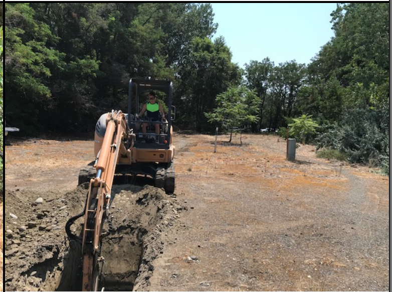
Excavation of test pit TP-8, view looking south
