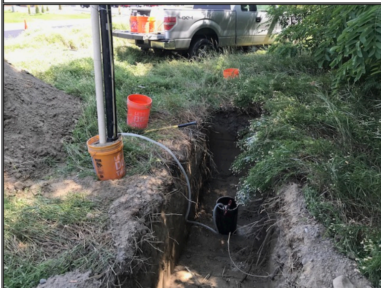
Infiltration test setup within test pit TP-10
