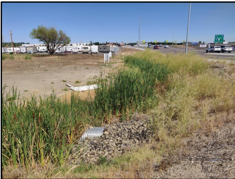
Typical City of Richland stormwater outfall (located west of the site)
